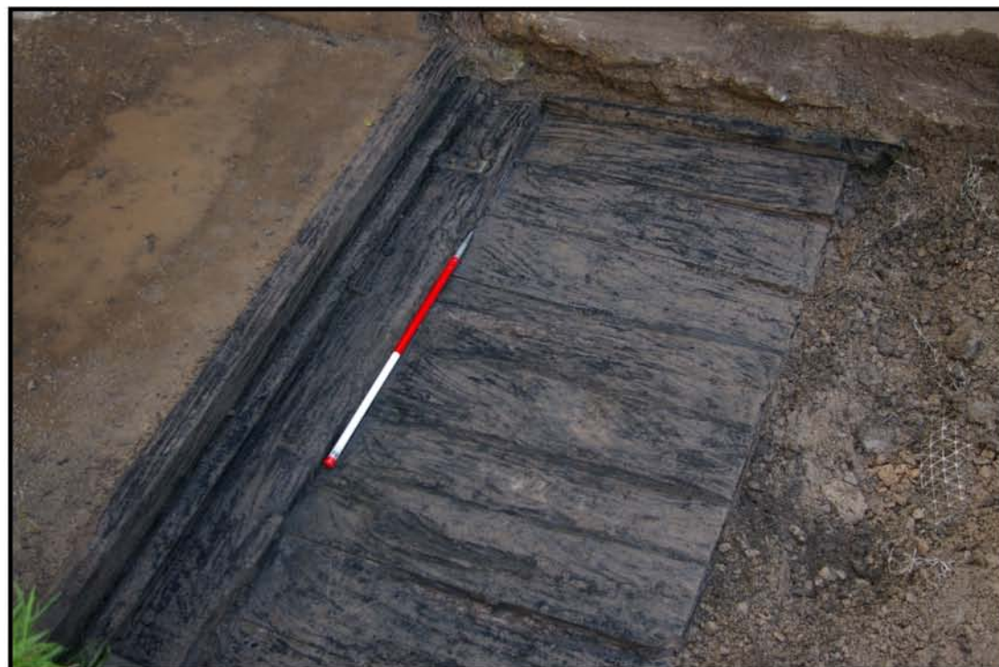
Fig 5: Lift gate in western forebay
