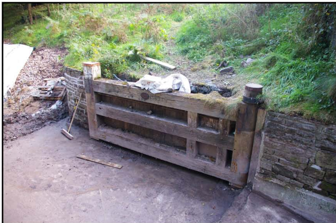
Fig 4: Swing gate in eastern forebay
